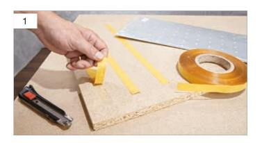
Place the particle board on two trestles and stick on pieces of double-sided tape. These will adhere better if you first use a hand brush to clear away any dust.
